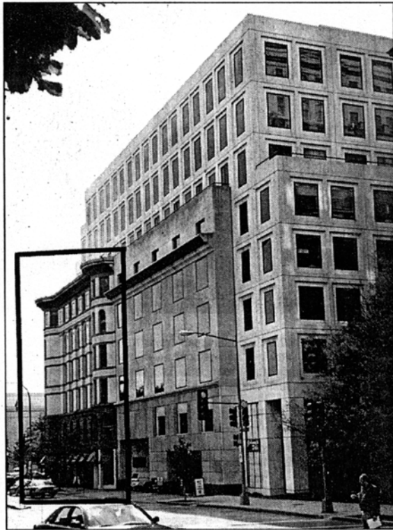
ABOVE: A black-line rectangle shows the original facade of the 19th-century Atlantic Coast Line building on the corner of Pennsylvania Avenue and Sixth Street in Washington, D.C., behind which a modern commercial building has been built. LEFT: A steel beam structure provides support for a facade with no building behind it. After the building is in place, the steel beams will come down.
