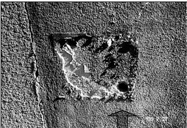
10.20. Location from which the left-hand plaque was removed from the Arch mural.
