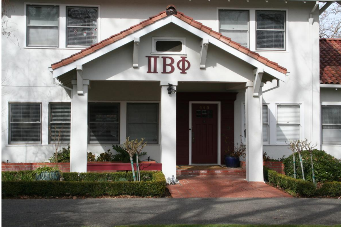
Photograph 4: Close-up of the south elevation of the house looking north. Note the original Craftsman front entry door.
