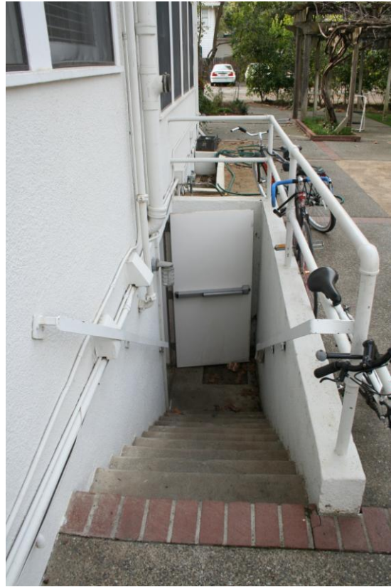
Photograph 19: View looking west down the concrete flight of stairs leading to the basement.
