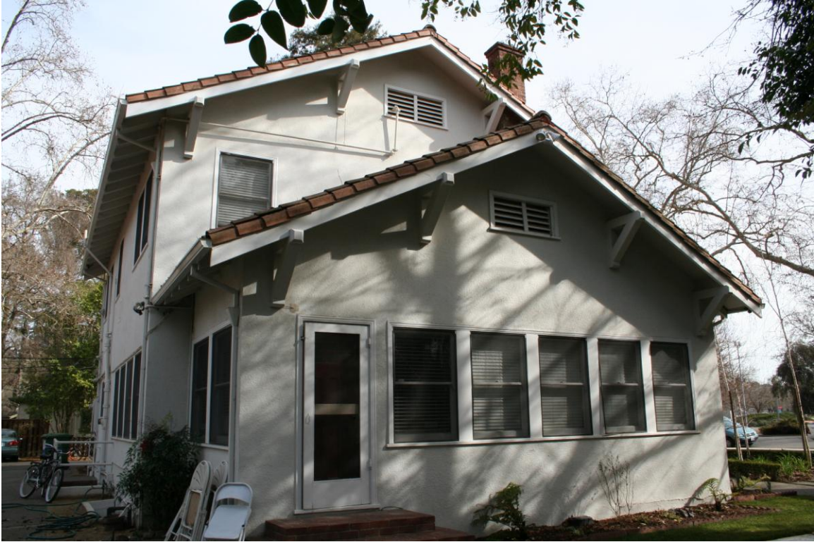
Photograph 7: View of the west elevation of the house. Note the original bank of double-hung, wood-sash windows and knee braces.
