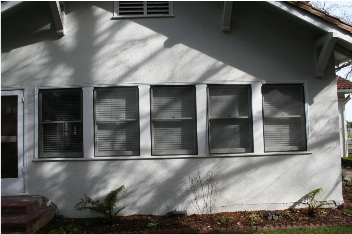
Photograph 8: Close-up of the window fenestration on the west elevation of the house.
