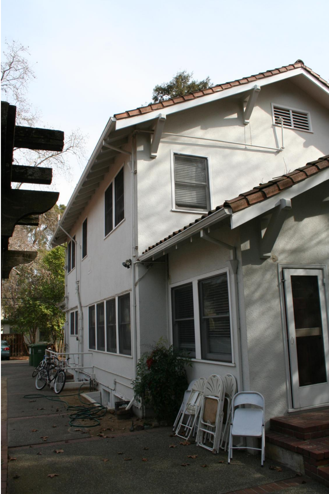
Photograph 9: View looking east at the north elevation of the house.
