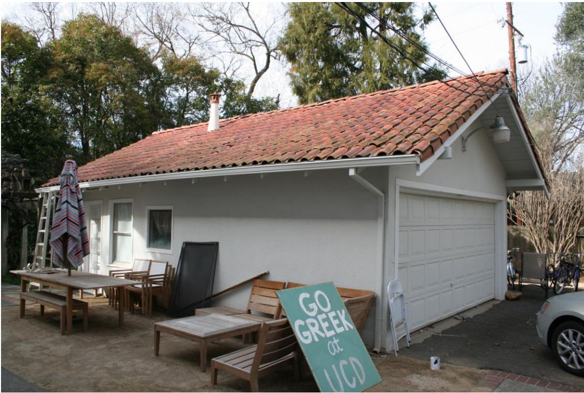
Photograph 13: View looking northwest at the southeast elevation of the garage.
