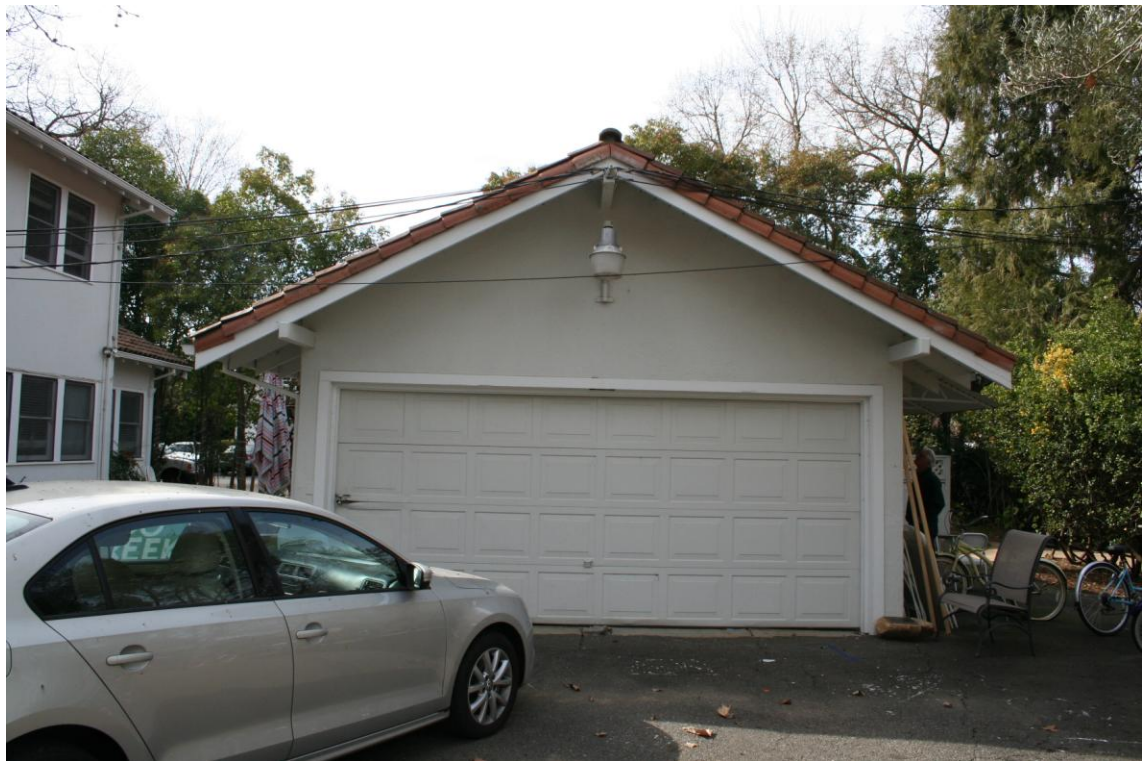
Photograph 11: Close-up of the replaced garage door.
