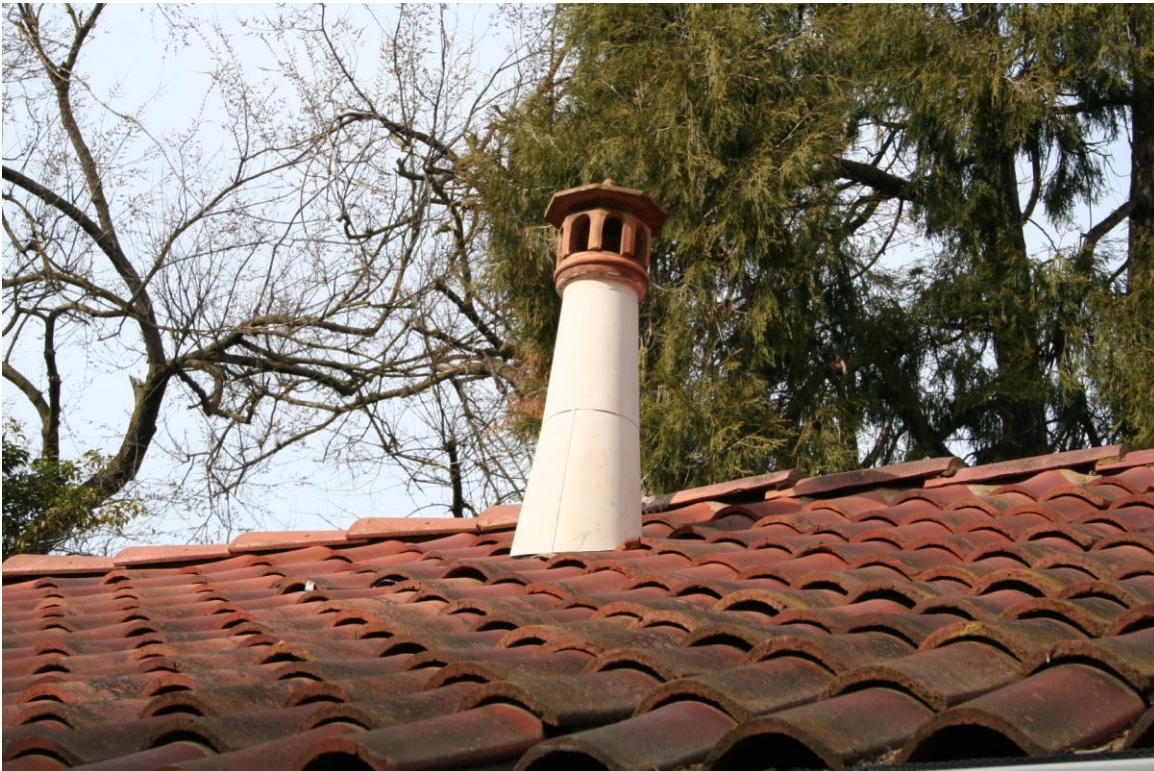
Photograph 15: View of the garage roof and decorative vent hood.
