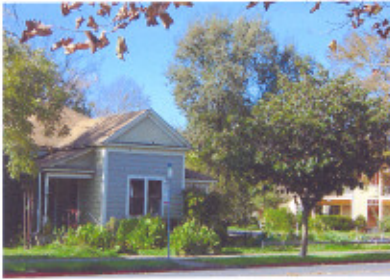
The McDonald House—337 B Street
