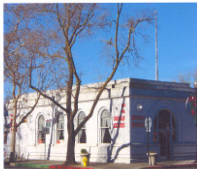
The Yolo Bank Building 301 G
