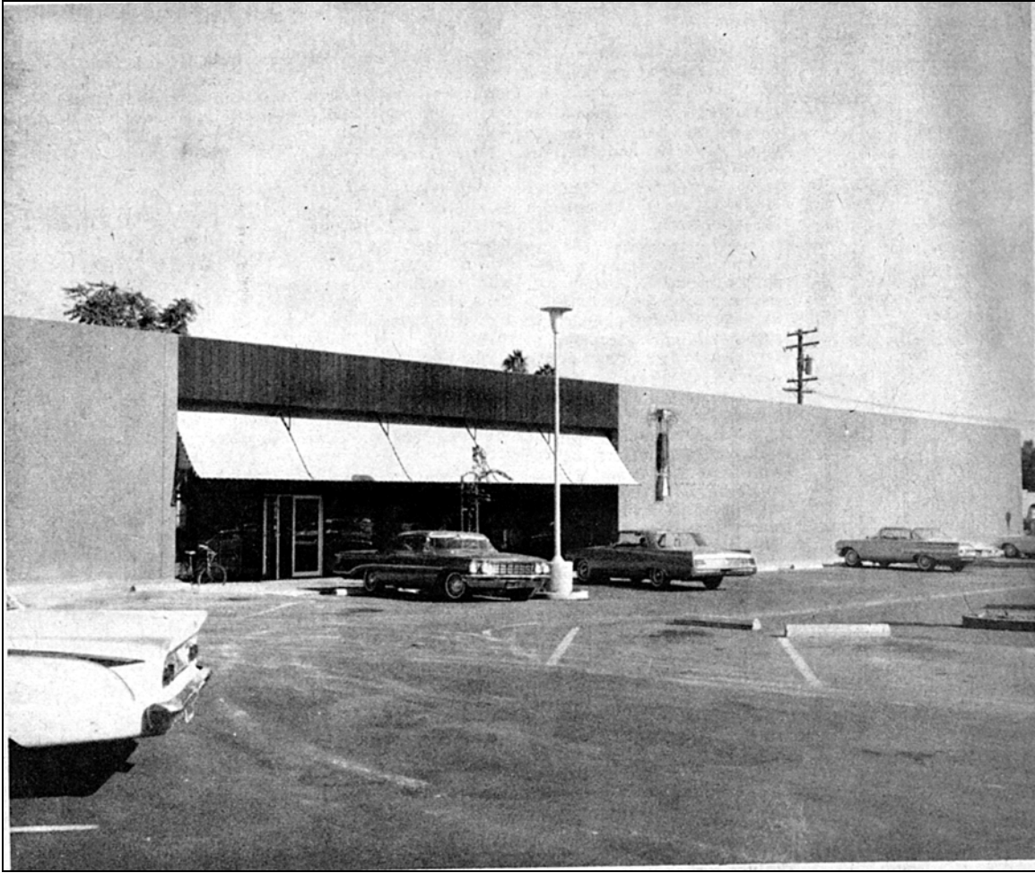
3.22. New Davis Lumber building, 1964. As can be inferred from image 3.21, just above (and from image 2.2.), the farther eastern part of the G Street block—which faces H street—is covered with sheds , not human-habitable buildings. These were the lumber-storage buildings of Davis Hardware and Lumber. Getting on the right side of history so to speak, this business removed that part of its operation and replaced it with the large hardware store shown here. Ever so conveniently, the building fronts the new parking lot. ( Davis Enterprise , December 4, 1964.)
