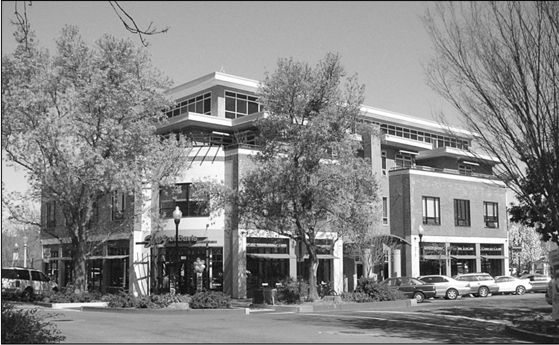
3.19. The Chen building on the site of the Terminal building, 2008. One major concern was that any new building not be out of scale with existing nearby commercial structures such as the Anderson Bank building. For this reason, the G Street facade of the new building is to the scale of the Terminal building and its third and fourth stories are seriously stepped back. (John Lofland.)
