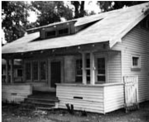
5.5. 618 F Street before renovation and remodeling. (Courtesy Roxie Eichelberger)
