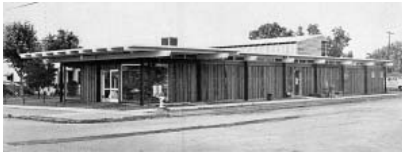
4.2. The Hibbert Lumber Company building in the late 1950s. There is no stop light or even stop sign at Fifth and G. Fifth Street ends at the railroad, just beyond the right edge of this photograph. (Courtesy Becky Hibbert)
