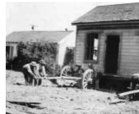
6.14. The original 618 E being moved, in the mid-1930s, from the block that will become Central Park. (Courtesy Helen Rowe)
