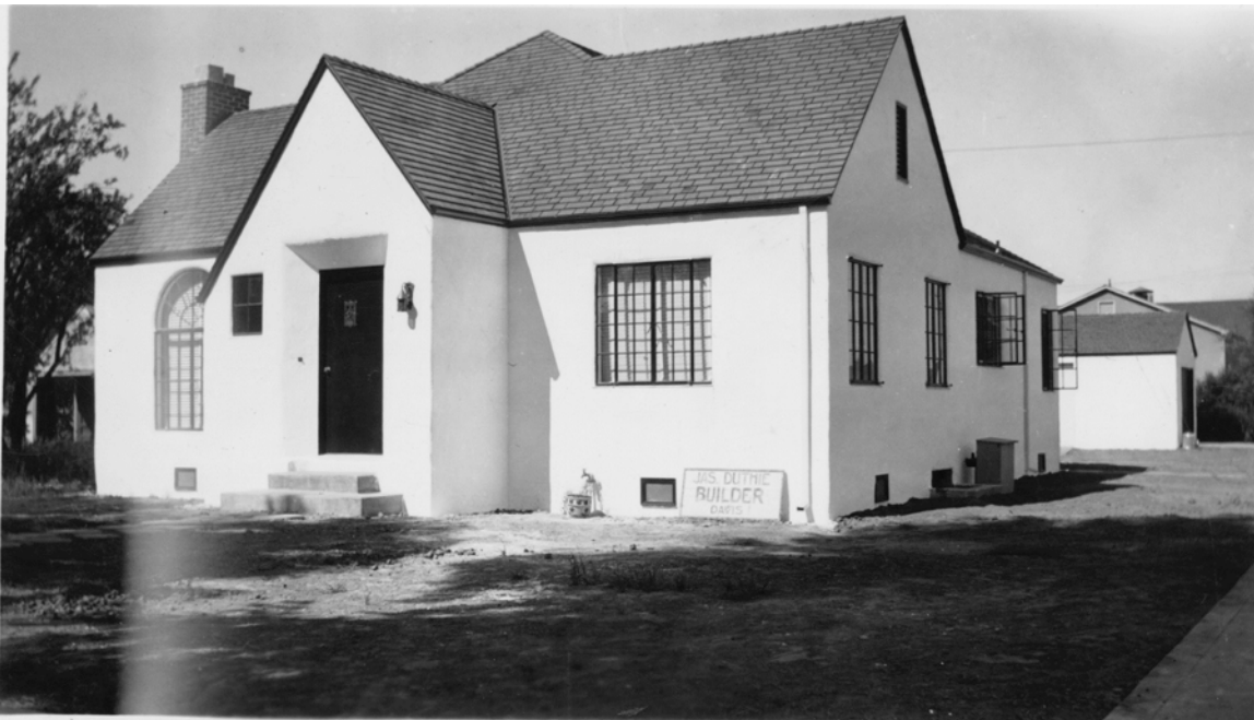
Two views under construction. Sign reads James Duthie the builder. Duthie lived in the next block up E Street.
