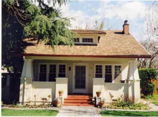
Classic Craftsman bungalow: full-width front porch formed by an overhanging roof, solid porch supports, one-and-a-half stories, hipped roof. (633 E)
