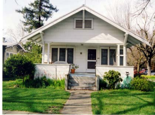
Front gable bungalow. (647 F)
