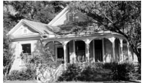
5.10. 623 Seventh Street, The Anderson- Hamel House.
