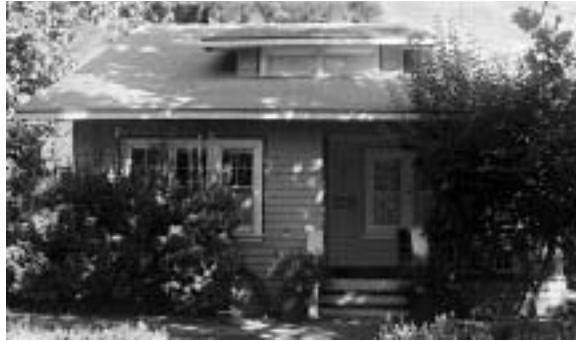
5.4. 618 F Street in the late 1990s, after renovation and remodeling.
